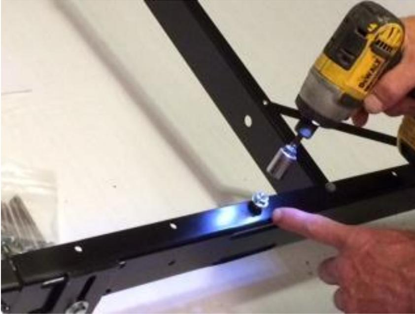
Each rack comes with a pre placed anchor spot for the inverters, with a bolt provided in position, although this bolt can be moved to any predrilled location in the main rail, 1<sup>st</sup> loosen the bolt
