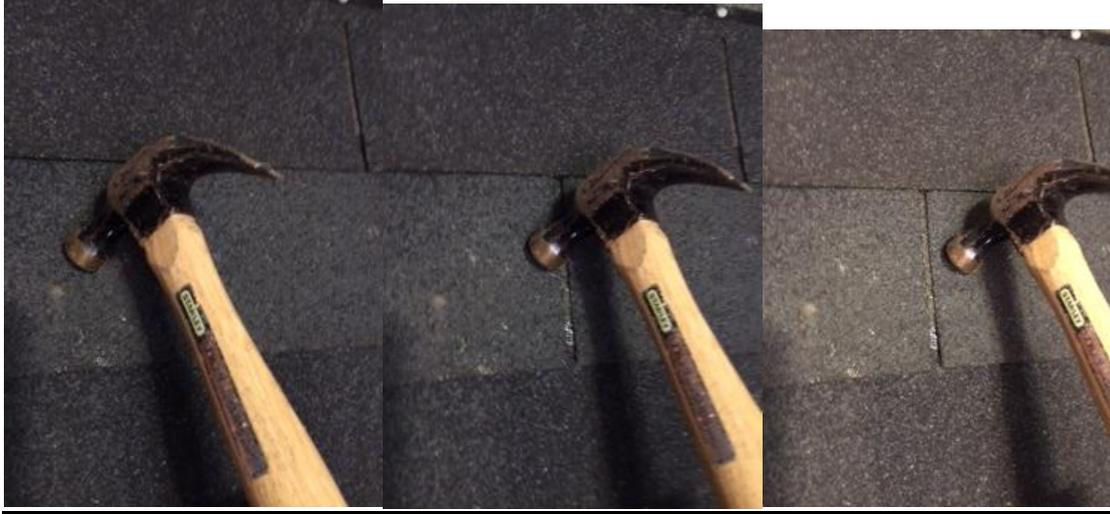
An industry standard way to locate roof rafters is to utilize a hammer and strike the roof while listening for sound differences, once the rafter location is determined a predrilled 1/4" hole should be made
