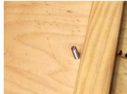
Confirmation of roof rafter can be determined by looking up at the roof rafters to determine if any Solar Lag bolts have “missed” the roof rafters
