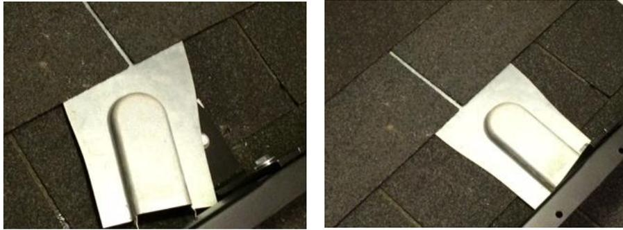
Continue to rotate the flashing under the shingle line until it is fully seated over the anchor foot
