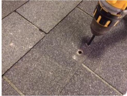
If the rafter is missed, small adjustments can be made to properly locate the rafter, these small adjustments will be protected by the anchor foot flashing to be installed later
